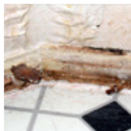
Mushrooms growing at the base of and behind the baseboard below a water leak in a bathroom. The baseboard has been removed; the puckers in the paint are due to water damage. (photo, John Martyny, Ph.D.)
