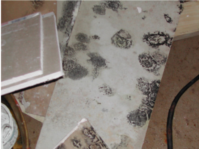
Mold on first floor beneath a through-the-wall air conditioner on the second floor. (photo, Terry Brennan)
