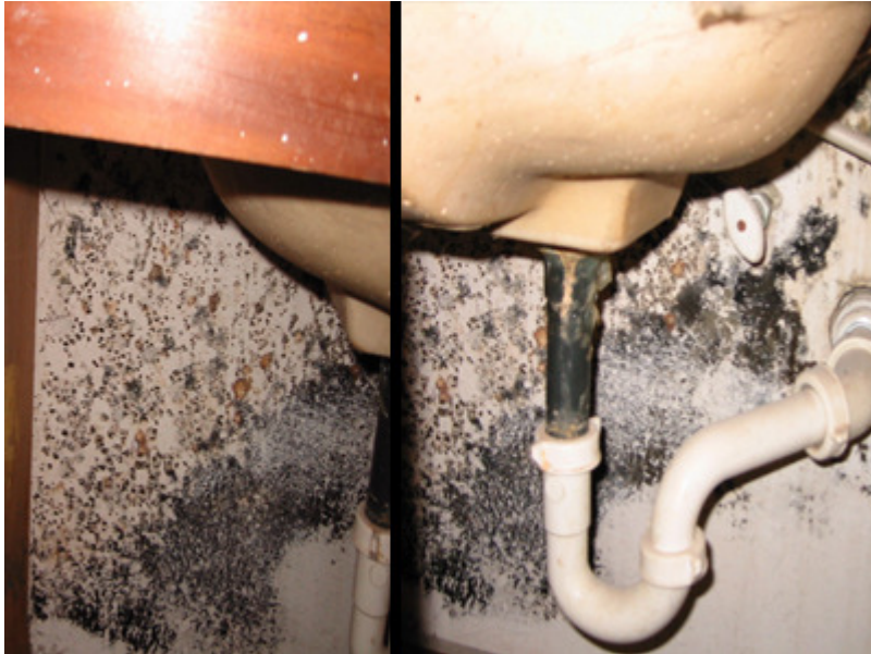
Plumbing leak inside wall led to mold on paneling behind mirror above bathroom sink. (The mirror has been removed in this photo.) (photo, S. McNeel, DVM)
