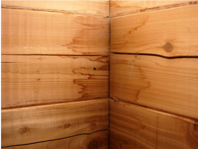
Water stains on wall and ceiling. (photo, John Martyny, Ph.D.)
