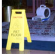
Drying a carpet with a commercial specialty blower with built-in heater. (photo, Terry Brennan)
