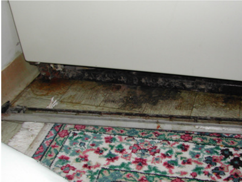
Mold on a vacuum cleaner stored in a damp basement. (photo, Terry Brennan)
