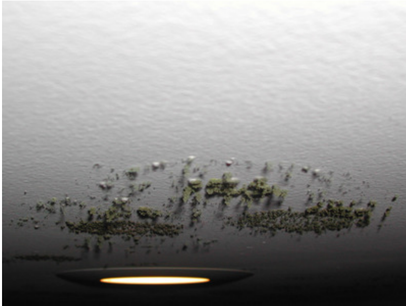
Mold on painted concrete in a school building. Rainwater is wicking directly through the concrete walls, and there is also condensation on the earth-chilled concrete (The floor is about 3 feet below ground level.) (photo, Terry Brennan)
